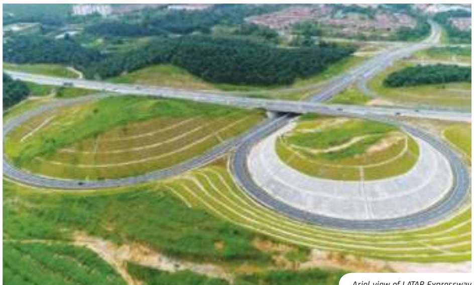
Aerial view of LATAR Expressway
